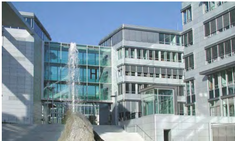
B/S/H company head quarters in Munich: Feng Shui and EnOcean radio systems under one roof
