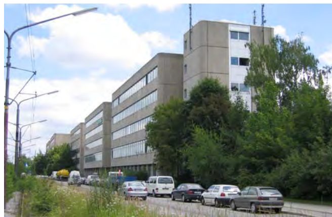
Siemens Munich: light and blind control in eleven office buildings using EnOcean radio sensors
