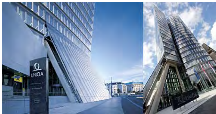
UNIQA company head offices in Vienna: EnOcean radio-based room sensors on 22 floors
